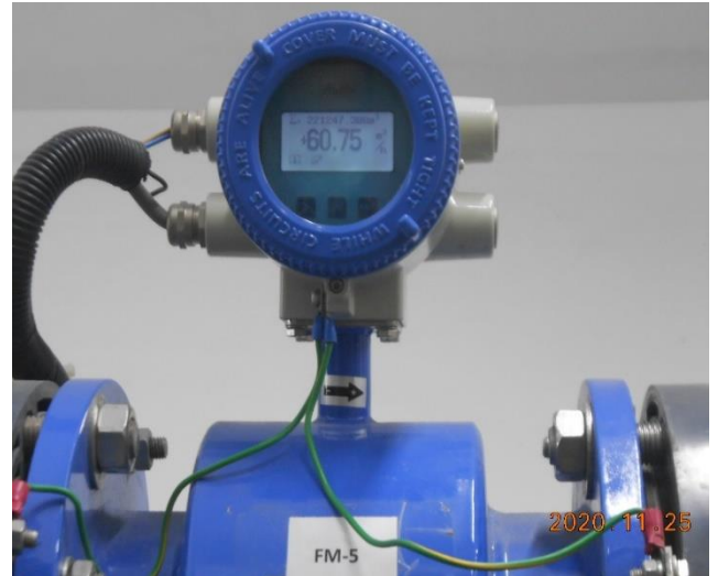
Water flow meter of wastewater treatment plant
